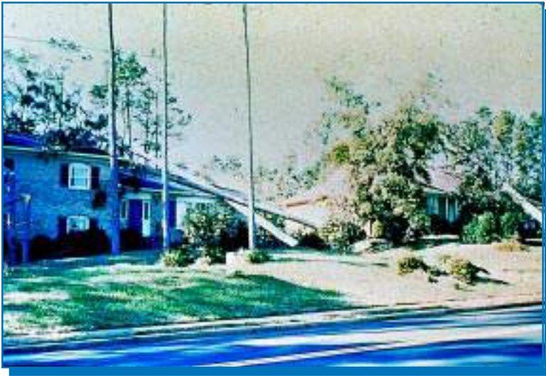
Hurricane Hugo wind damage, Charlotte, NC/NOAA
